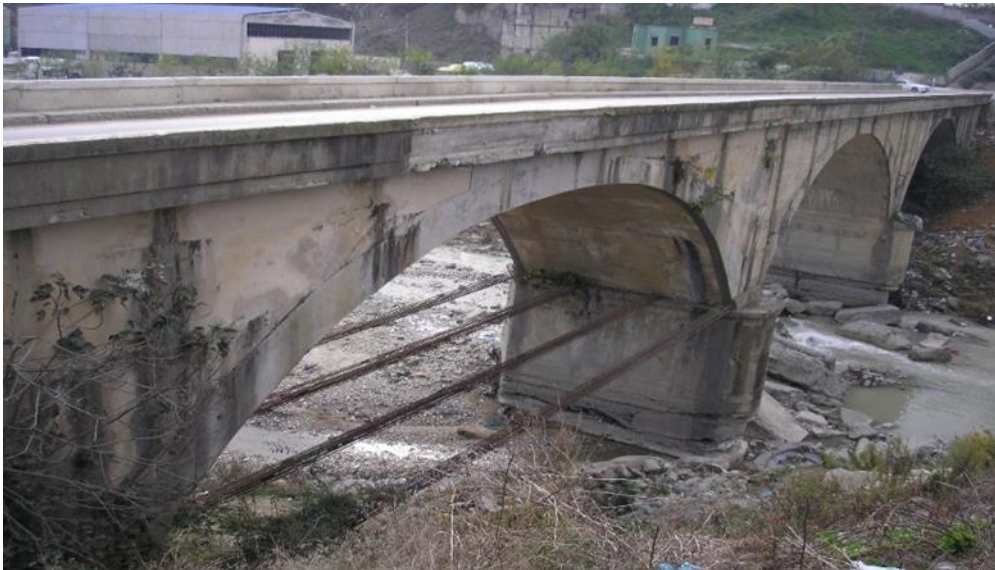
Beshiri Bridge over the Erzeni River – longitudinal view
